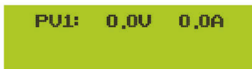
Pic 8.3 PV input voltage and current information
