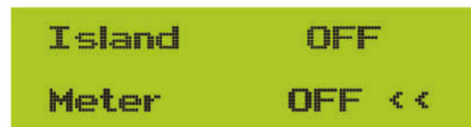
Pic 7.4 Meter switch
